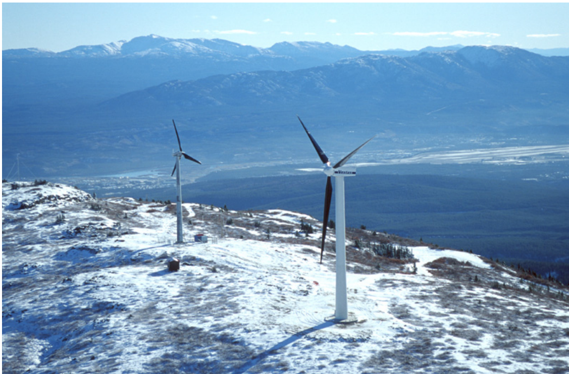
Photograph 10: both wind turbines in place
