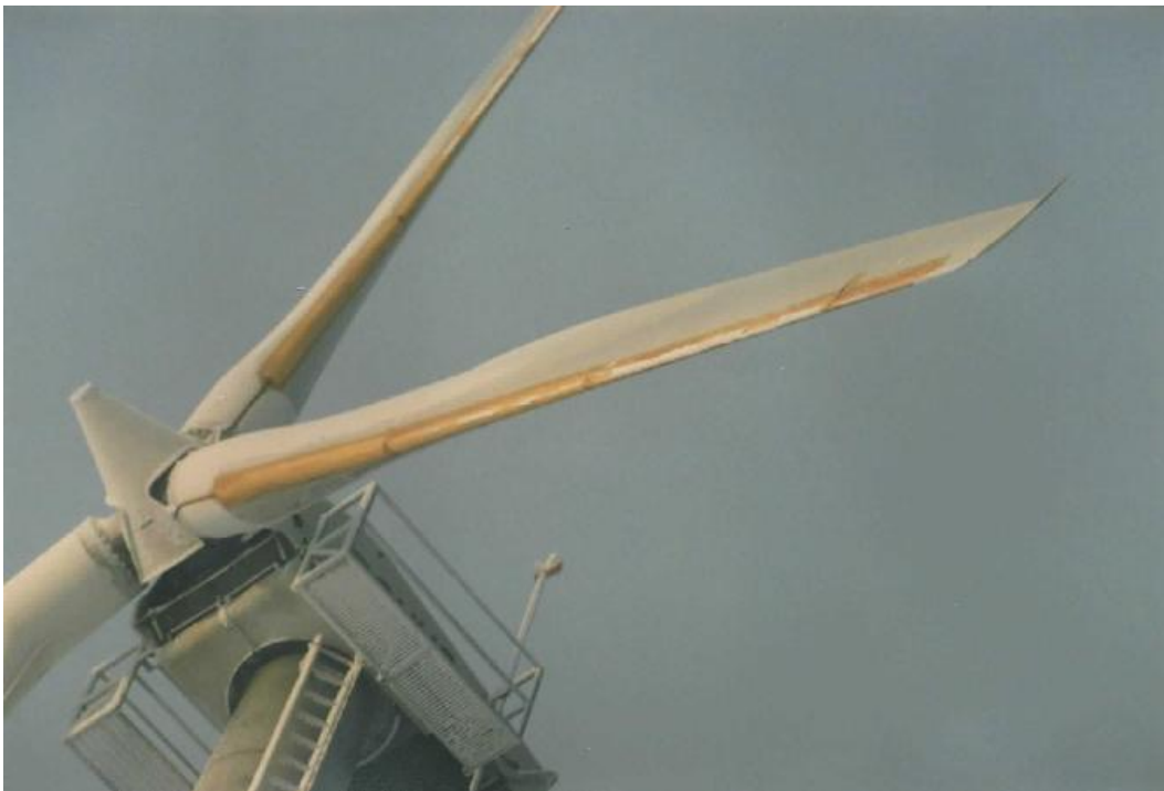
Photograph 6: in less severe rime icing the effect of the leading edge heaters extends past the leading edge
