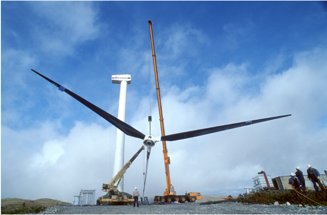
Photograph 9: the second wind turbine being installed
