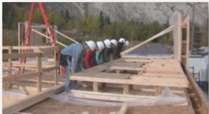
Figure 4: Larsen wall-truss system
