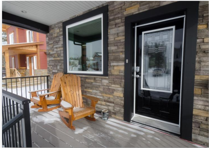
Figure 4: Window and exterior door
