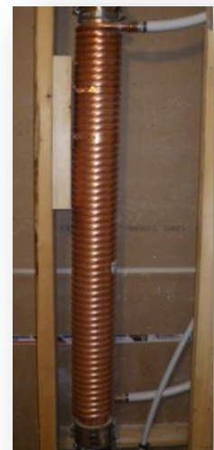
Figure 4: Drain water heat recovery
