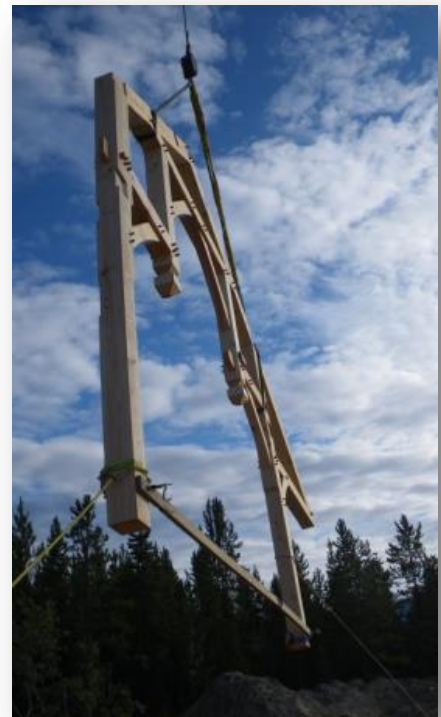
Figure 2: Setting timber structure
